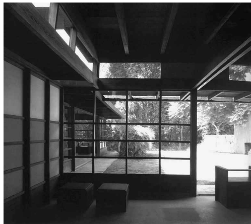
Figure 14. Frame construction in Pauline Schindler's studio. Photograph by Grant Mumford.
