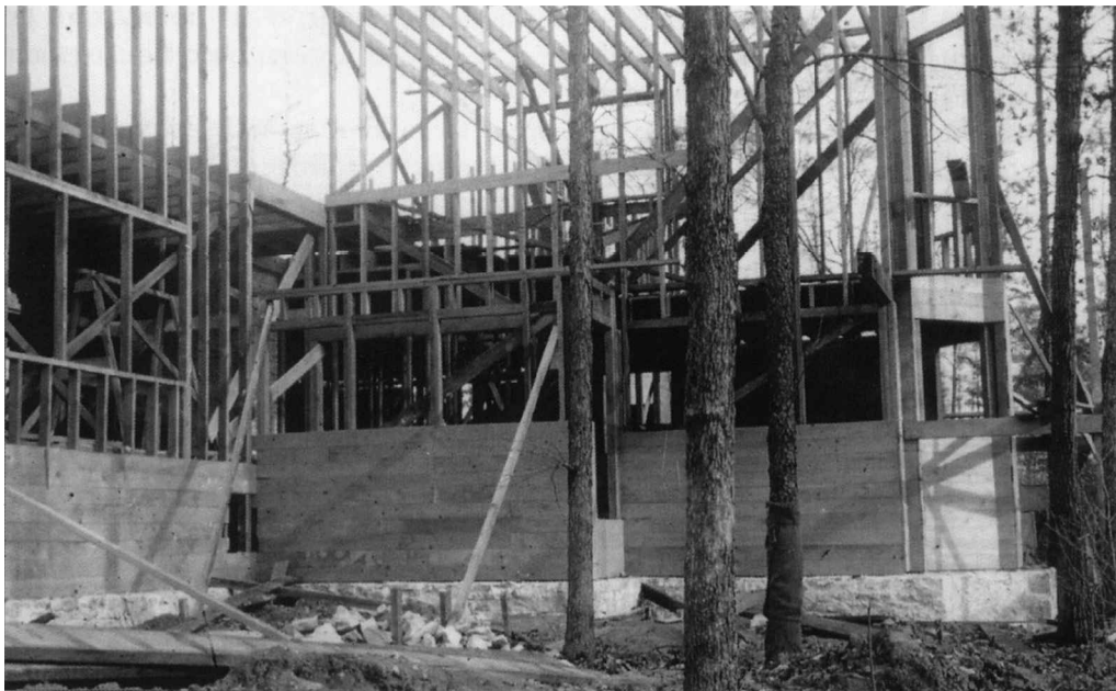
Figure 2. Ward Willits house 1901, balloon frame construction. The Frank Lloyd Wright Foundation.
